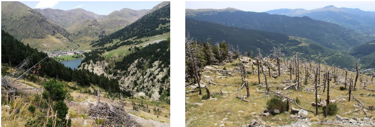
Figure 6. Núria valley. Avalanche transit area affecting the train railway which is protected with defensive infrastructures and a protocol of controlled avalanche trigger (left). Area affected by 2007 wildfire of Queralbs (right).
